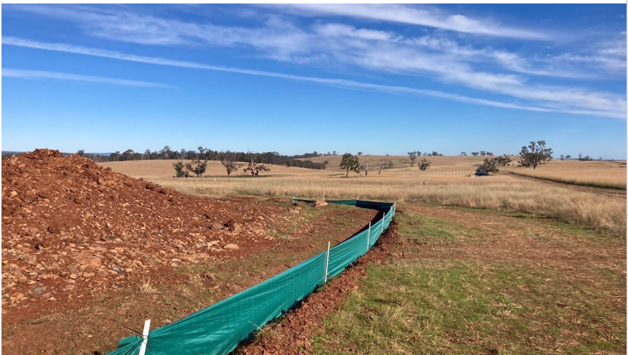
Transgrid pad earthworks ERSER controls
