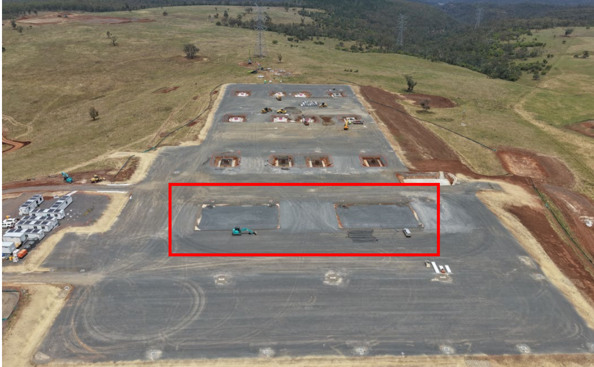
Figure 1. Transformer bund location on the substation bench
