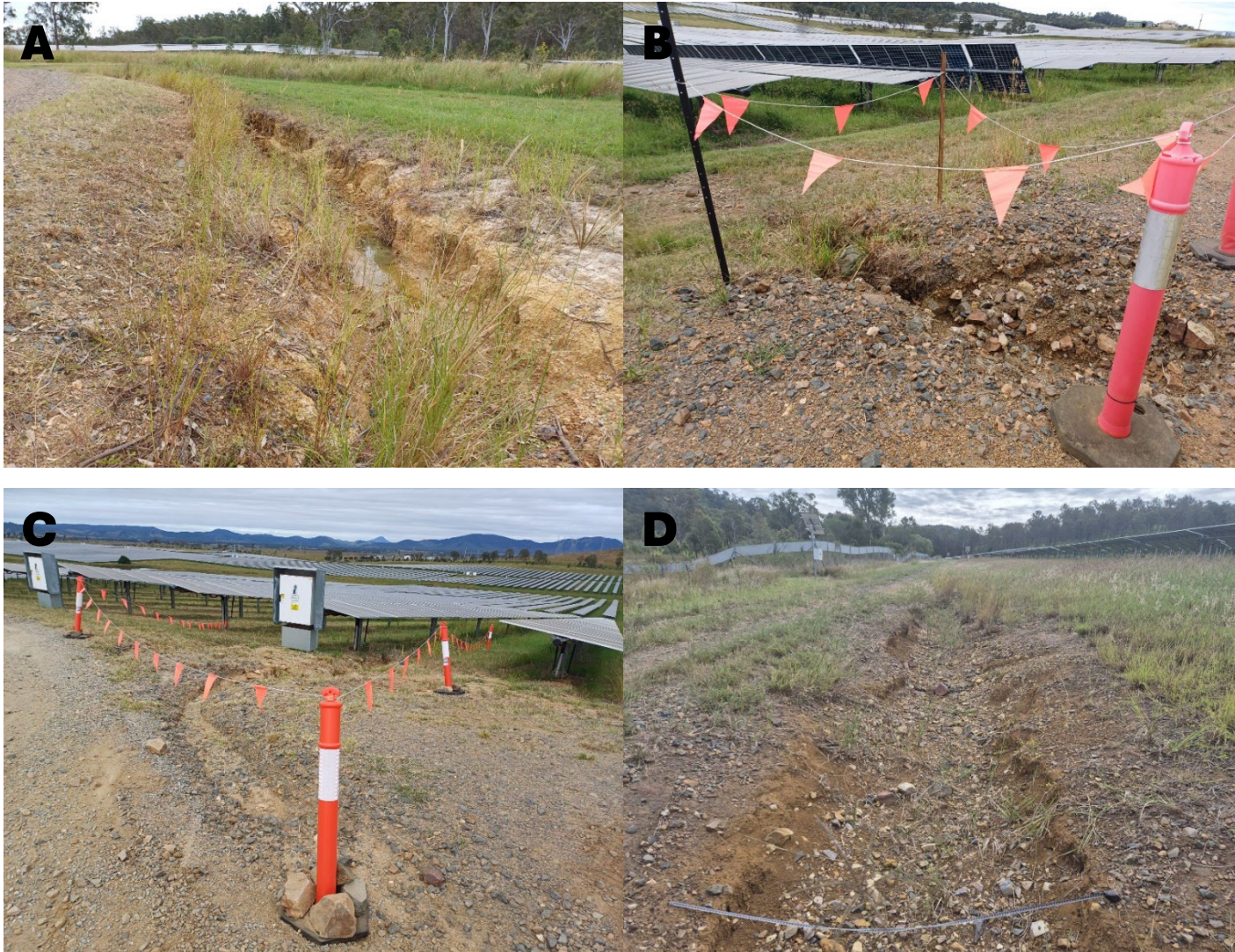
Woolooga Solar Farm, Lower Wonga, Queensland (EPBC 2019/8554)
