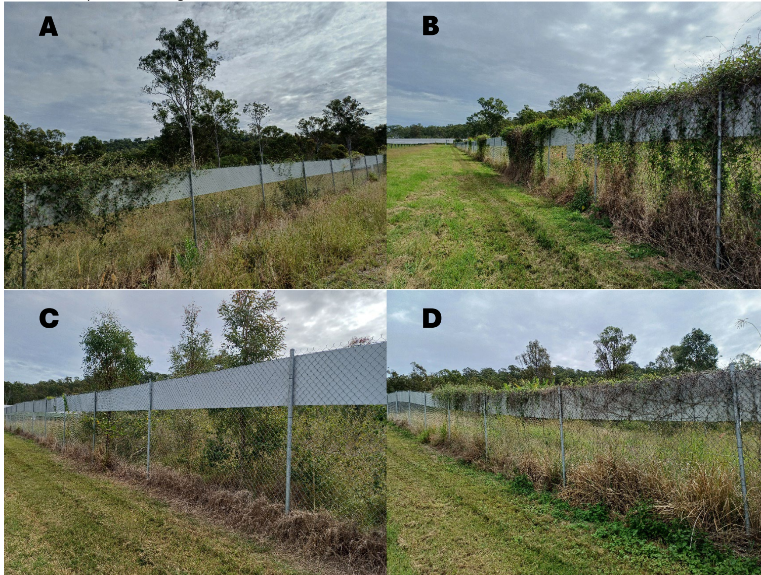
Woolooga Solar Farm, Lower Wonga, Queensland (EPBC 2019/8554)
