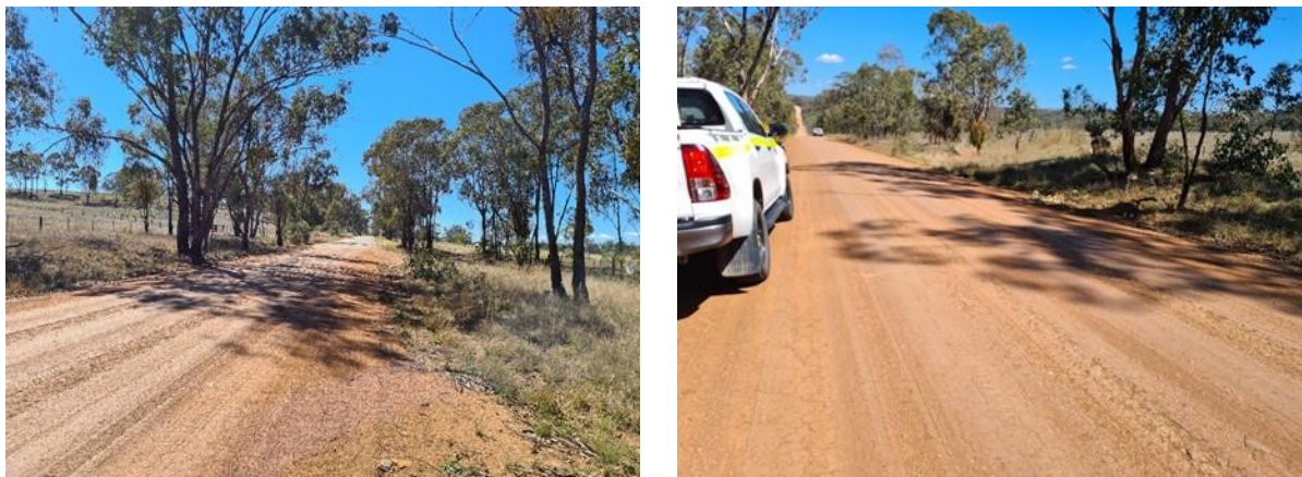
Figure 2-5: Wollara Road looking north (left) and south (right)
