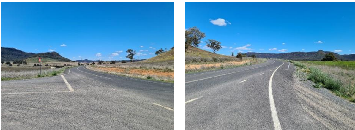
Figure 2-6: Wollar Road looking east (left) and west (right)
