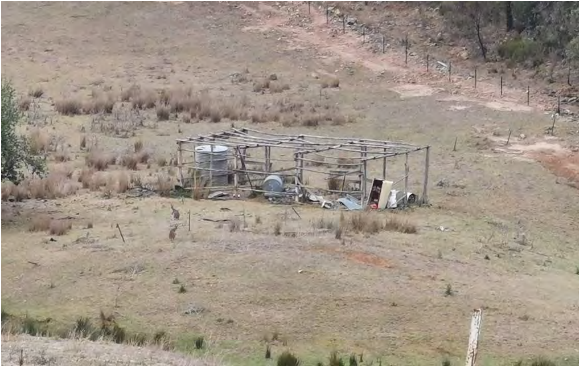
Photo 6.7 Partially dismantled shed located within the Development Footprint near Redlynch Creek
