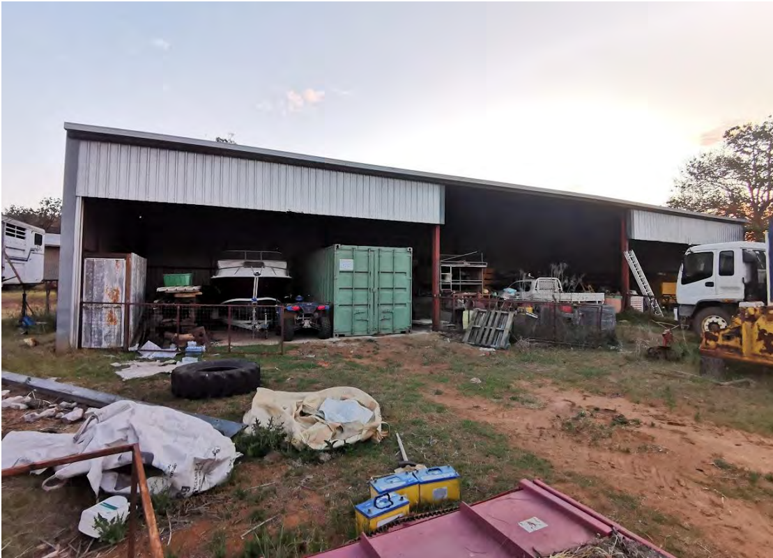
Photo 6.3 Operational open farm shed located within the Development Footprint
