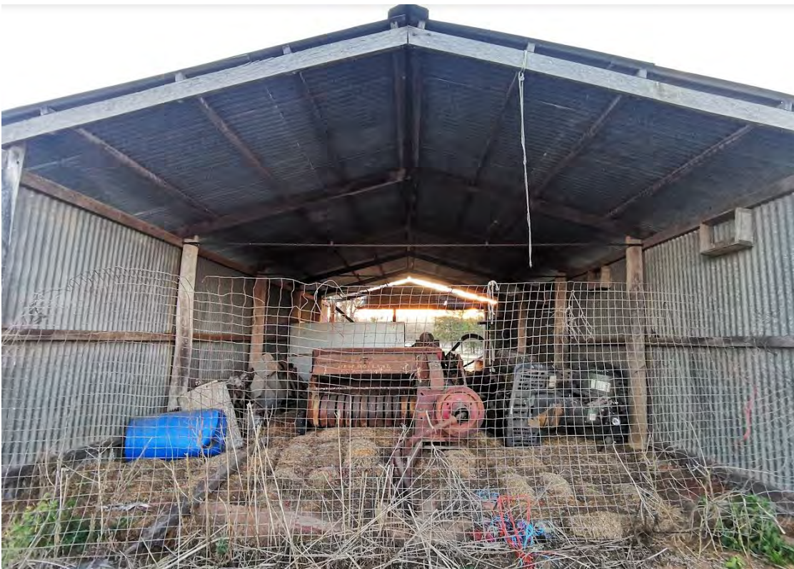
Photo 6.2 Operational open farm shed located within the Development Footprint
