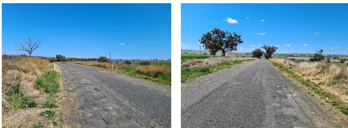
Figure 2-4: Ringwood Road looking south (left) and north (right)
