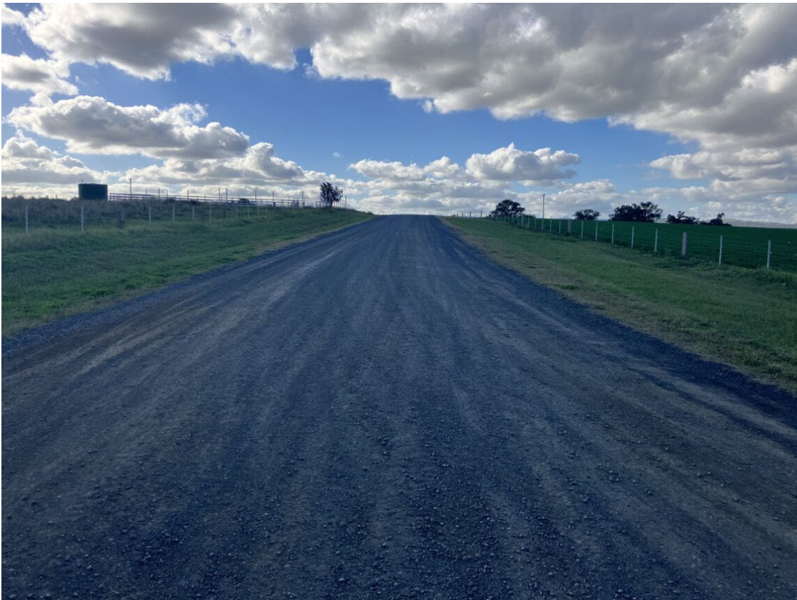
Photo 3.3 Typical vegetation either side of the Barnett Street road upgrades area
