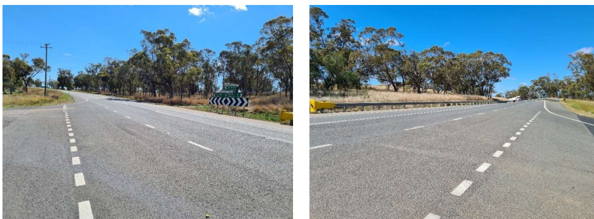
Figure 2-3: Golden Highway looking west (left) and east (right)
