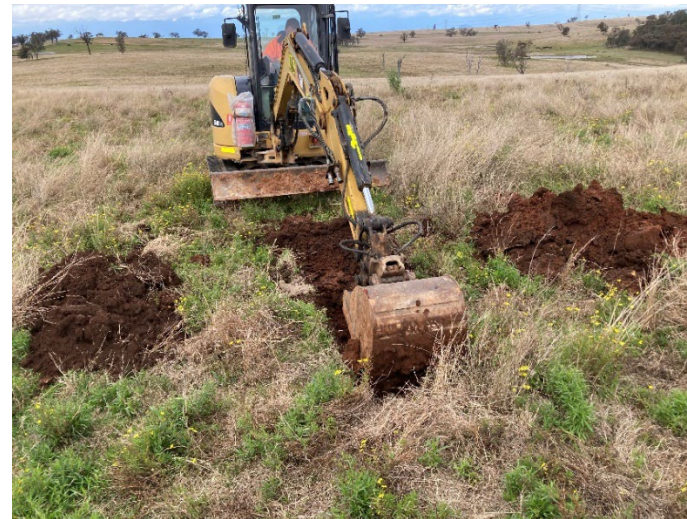
Photo 20 – Excavated soil material
