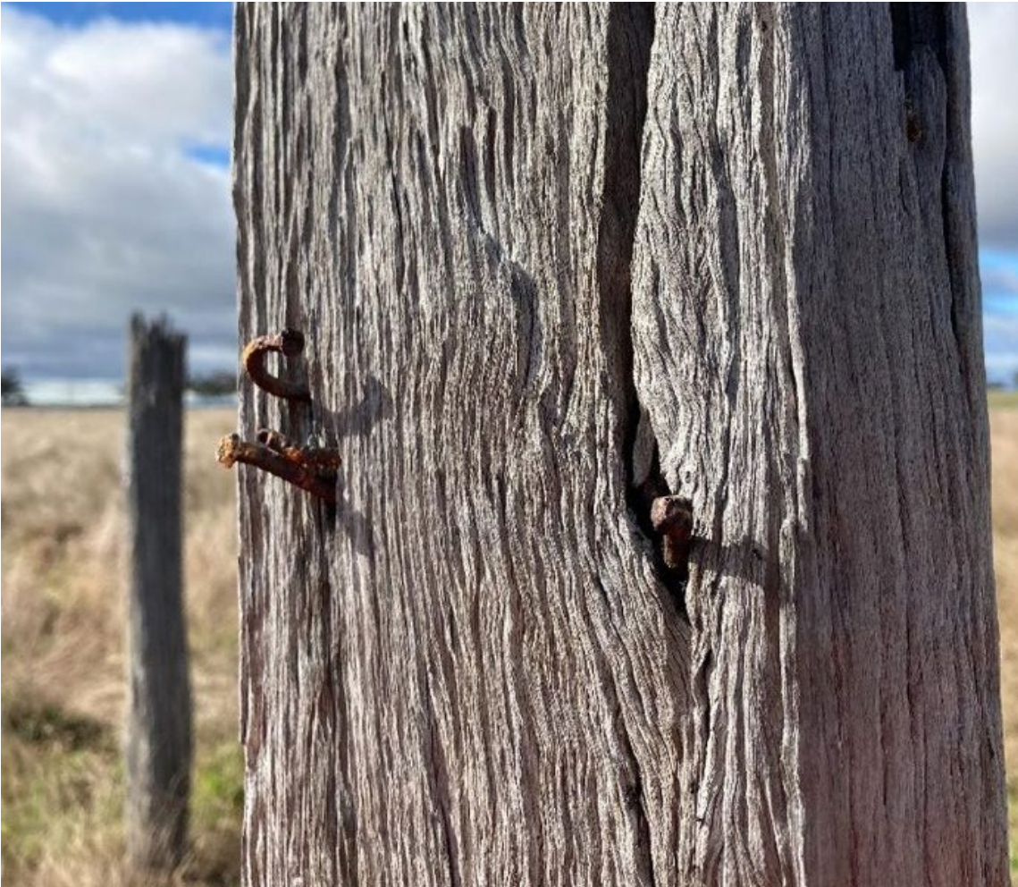
Photo 4.17 In-situ hand forged nails, note the warped form (Slab Hut)
