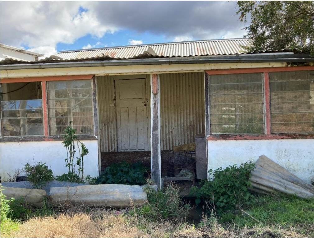
Photo 4.7 Southern enclosed portion of the dwelling (1900 house)
