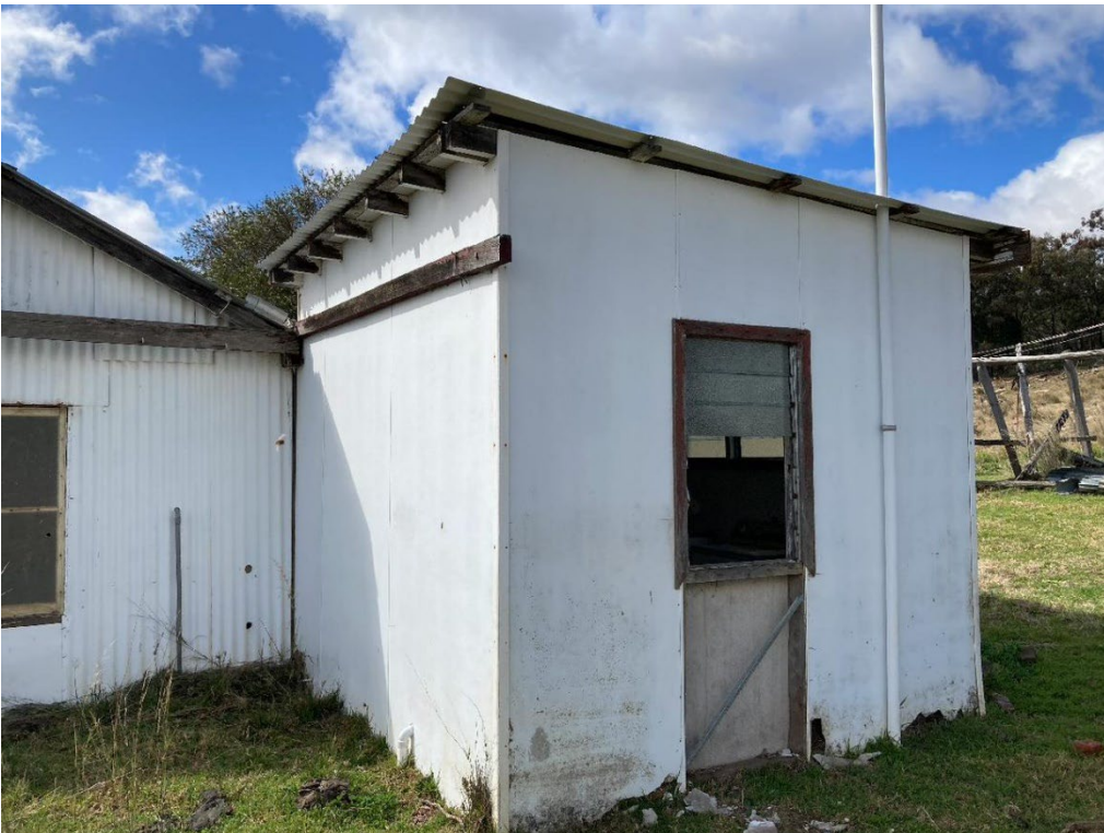
Photo 4.8 Mid 20th century bathroom extension (1900 house)
