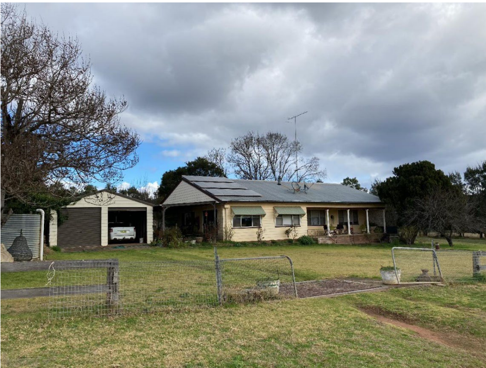
Photo 4.2 Primary residential dwelling (Post War House)
