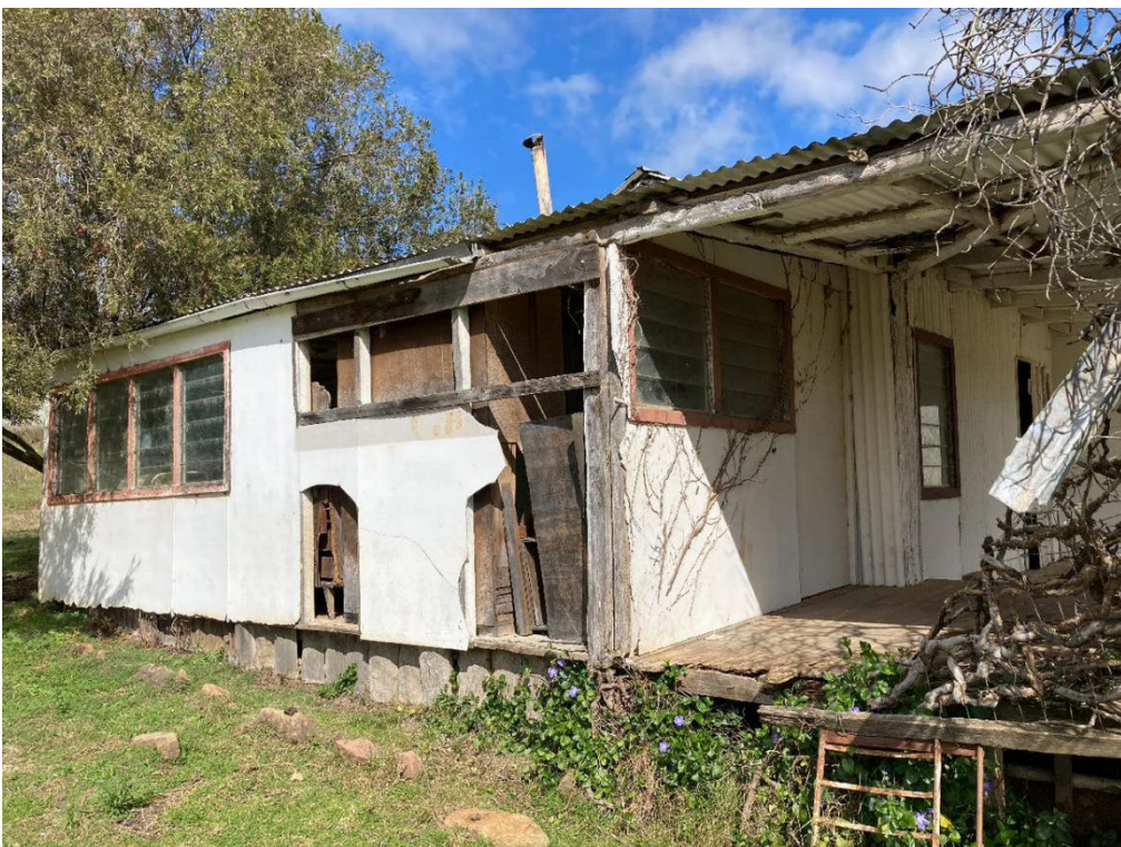
Photo 4.6 Materiality of the secondary dwelling (1900 house)
