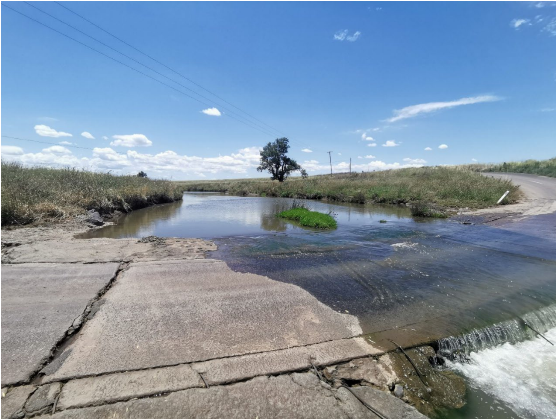
Photo 2.1 View of Bow River watercourse crossing looking upstream
