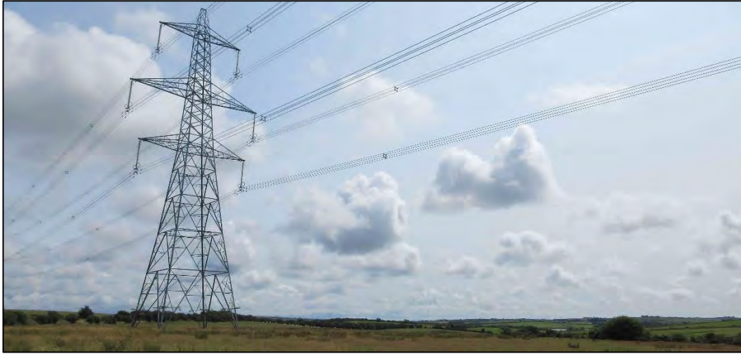
Photo. 17 Transmission tower within Maen Hir Central, viewed from the north-west
