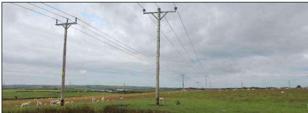
Photo. 16 Overhead powerlines within Maen Hir North, viewed from the north
