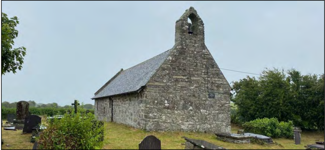
Photo 42 Church of St Pabo, viewed from the south-west
