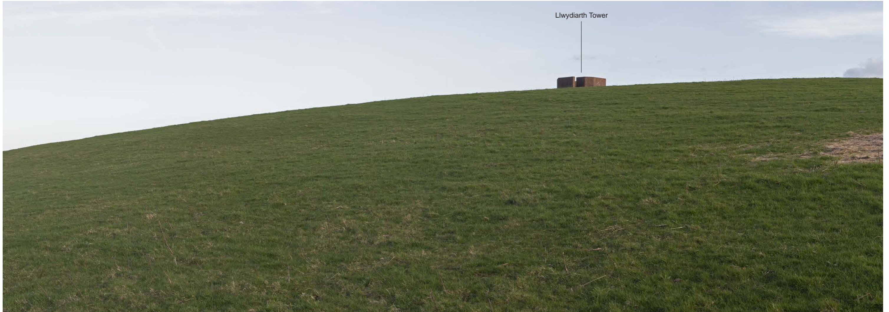
Representative Viewpoint 18 (Right Centre) - Public footpath LLANNERCH-Y-MEDD|25/002/1 near Pen-y-Foel and Llwydiarth Tower
