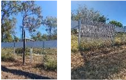
Plate 16 Fauna features on perimeter fence. Left photo shows koala pole crossings. Right photo evidence of a fauna grounding point.
