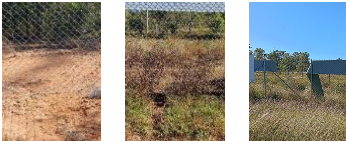
Plate 17 Fencing observations requiring corrective actions. Left photo evidence of a gaps between the fence and the ground. Middle photo evidence of a hole on the fence caused by fauna. Right photo evidence one loose exclusion fauna panel.
