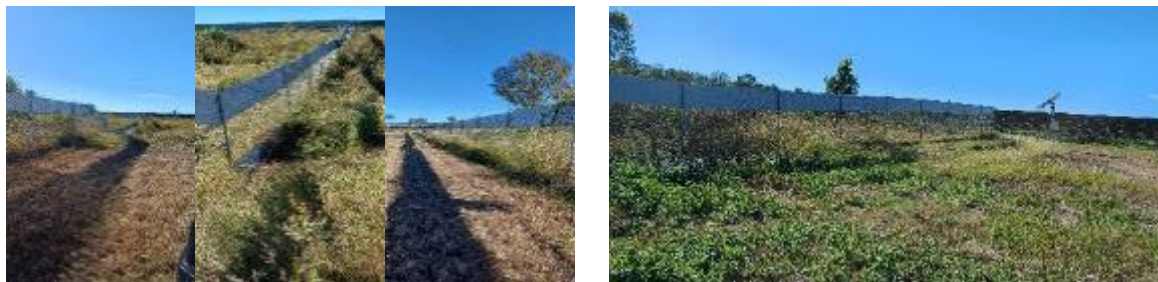
Plate 15 General good condition of the perimeter fencing. Photos show the koala exclusion panels along the northern boundary of the solar farm. Right photo shows evidence of effective corrective measures on previously reported fence damage (ACR1-Fence2).
