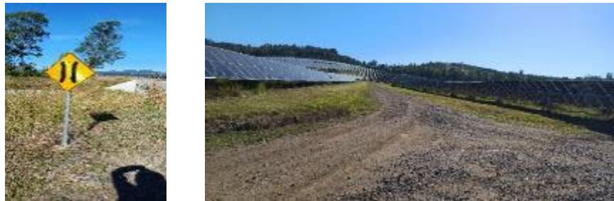
Plate 14 Traffic signalling within the solar farm premises. Left photo showing signalling at the waterway crossings. Right photo evidencing lack of speed limits or calming traffic measures on the roads.
