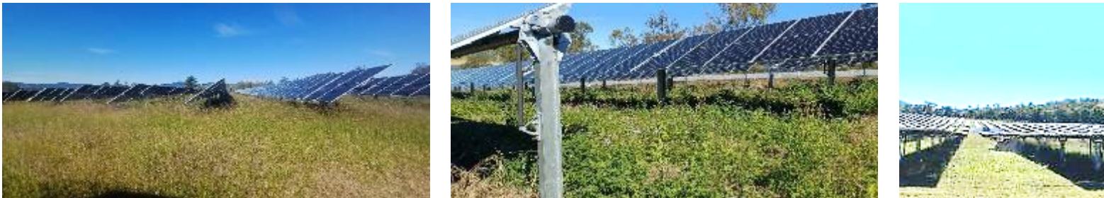
Plate 18 Weed management within the premises. Left photo evidence Chloris gayana overgrowth. Middle photo evidence billy goat weed overgrowth. Right photo shows ongoing maintenance works on site, consisting of mowing vegetation below panels.
