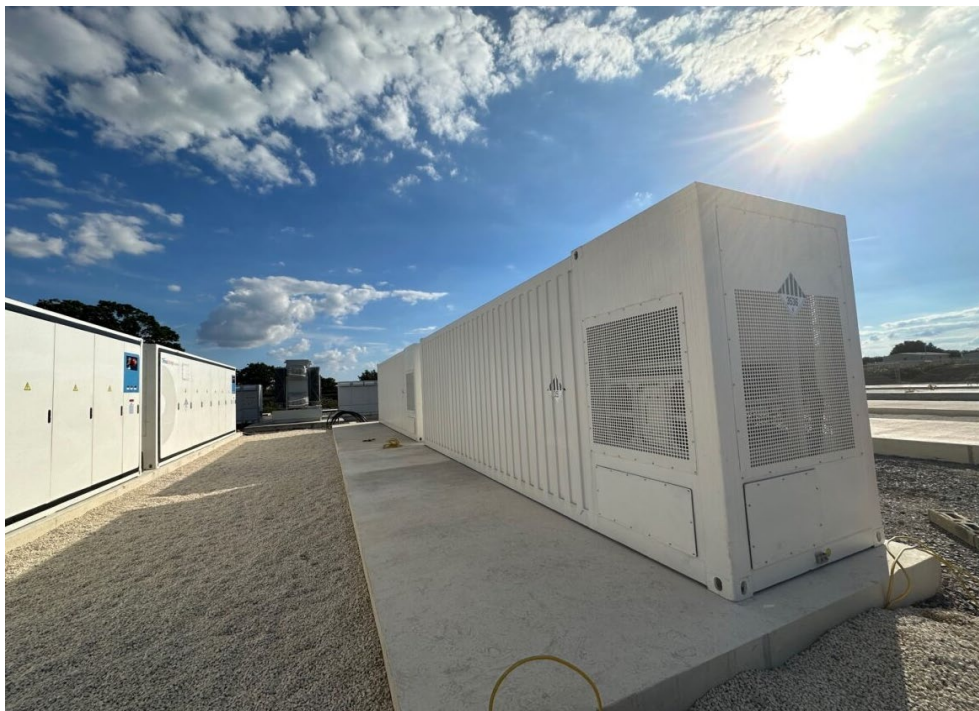
Figure 7: BESS Enclosure - Lightsource bp site at Tilm, Nottinghamshire during construction
