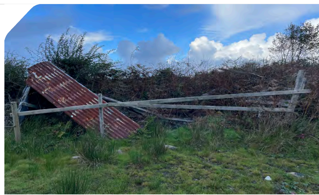
Plate 14: Field 3 – W Facing – Dilapidated Barn Structure
