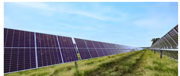
Solar panels are mounted on posts, enabling growth of vegetation underneath that allows for natural drainage and the interception of storm water
