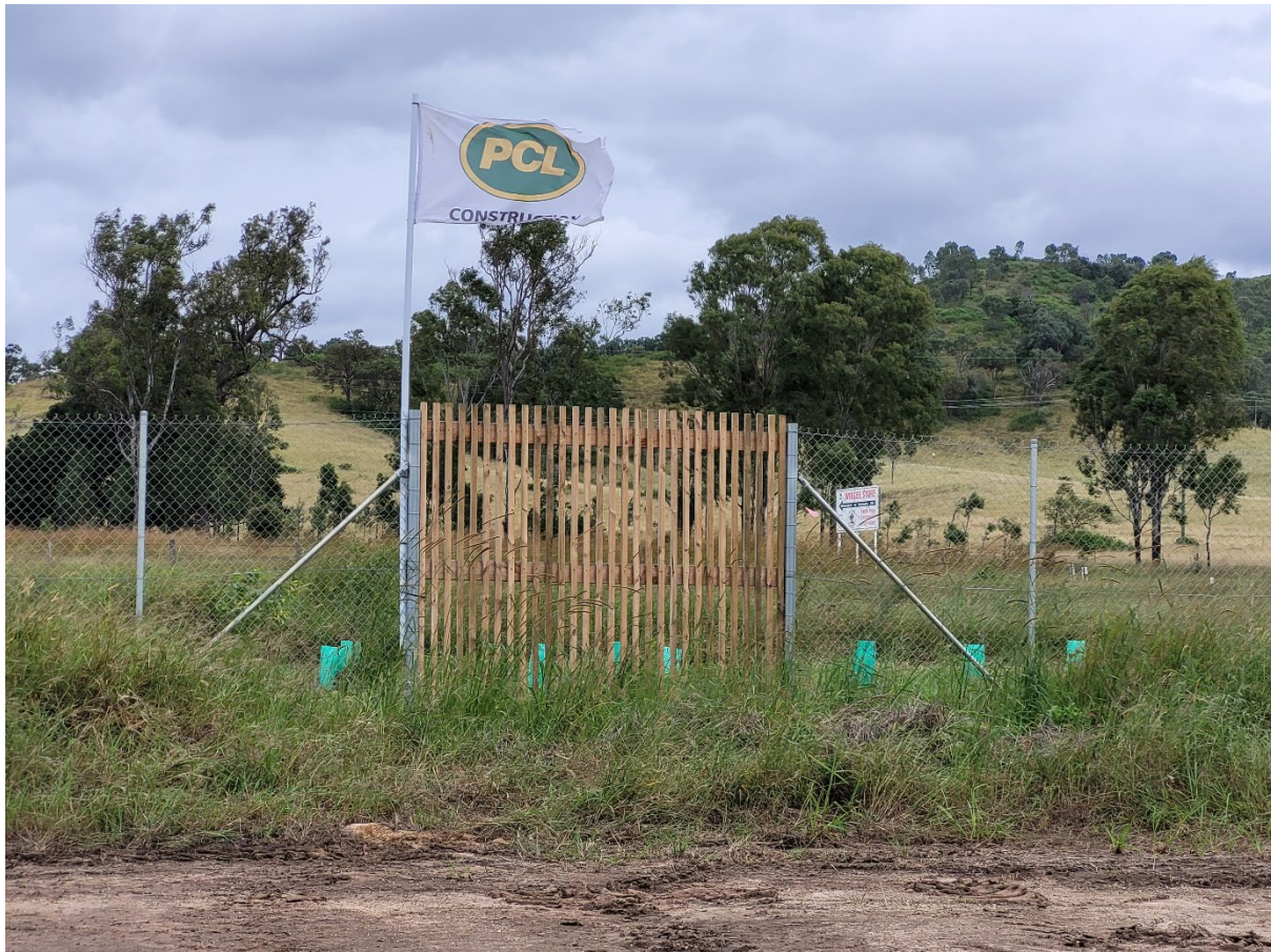
Photo plate 41; an image of a fauna grounding point located on the southern boundary fence nearby to culvert 9
