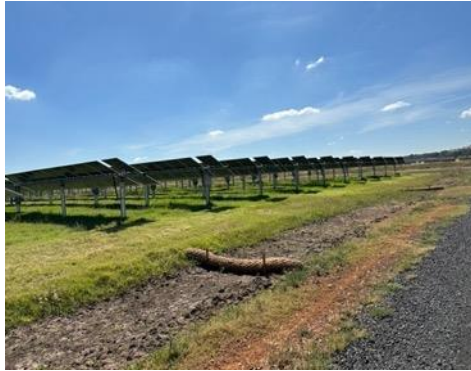
Photo 17: Evidence of erosion and sediment control fencing used in key drainage area on site.
