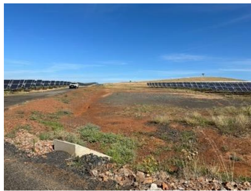
Photo 4: Internal drainage lines with culverts.
