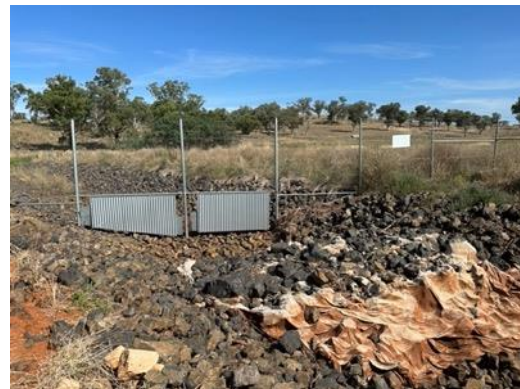
Photo 12: Perimeter gate with moveable storm flow barrier.
