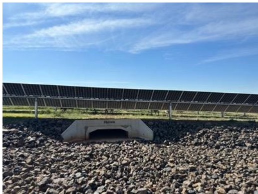
Photo 11: Example of rock lined drainage channel and under array culvert.
