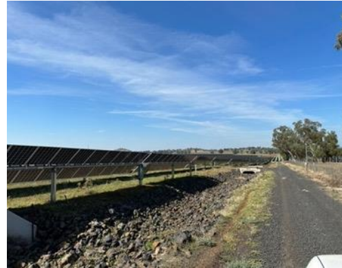
Photo 10: Perimeter road and rock lined dish draining channel.
