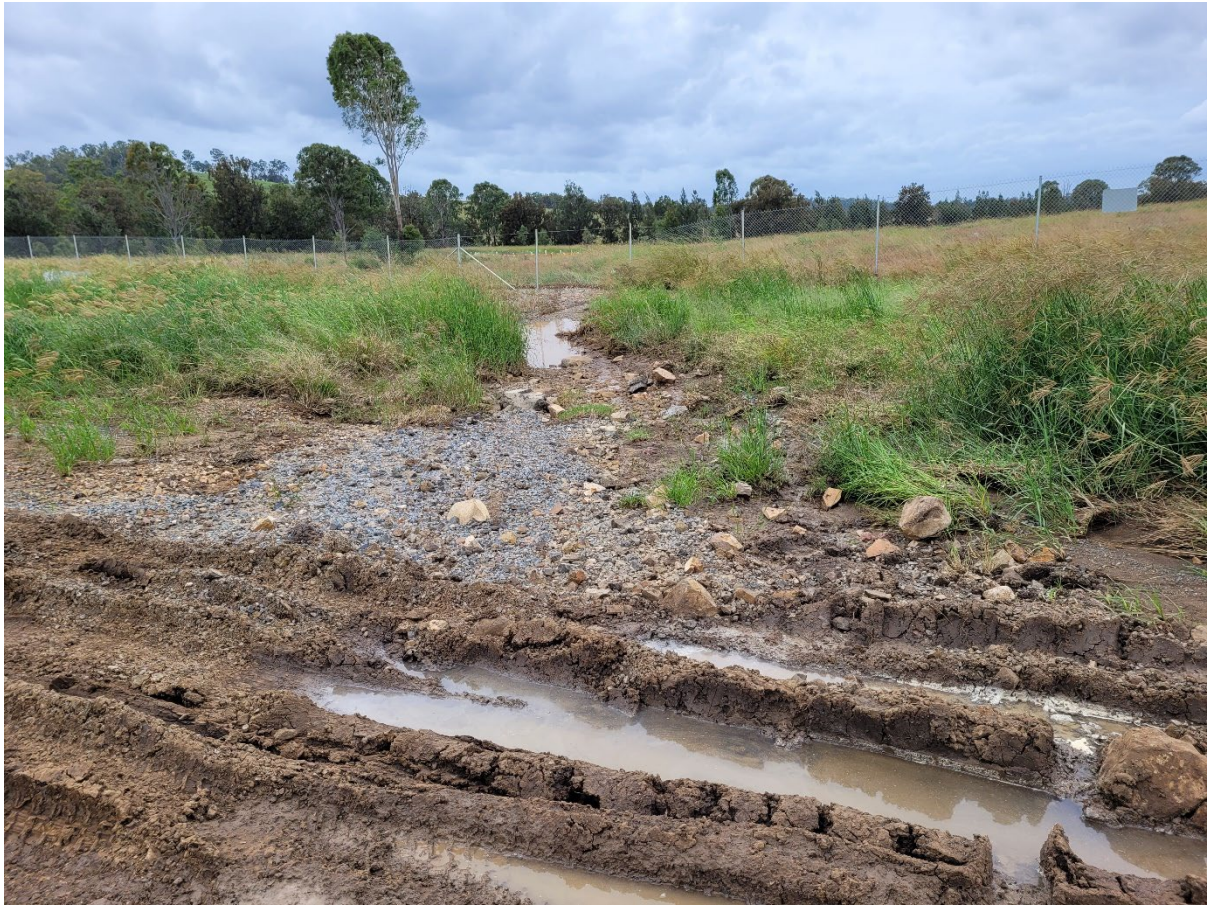
Photo plate 12; a photo of the downstream side of culvert 1, taken facing east showing the movement of sediment towards the boundary fence
