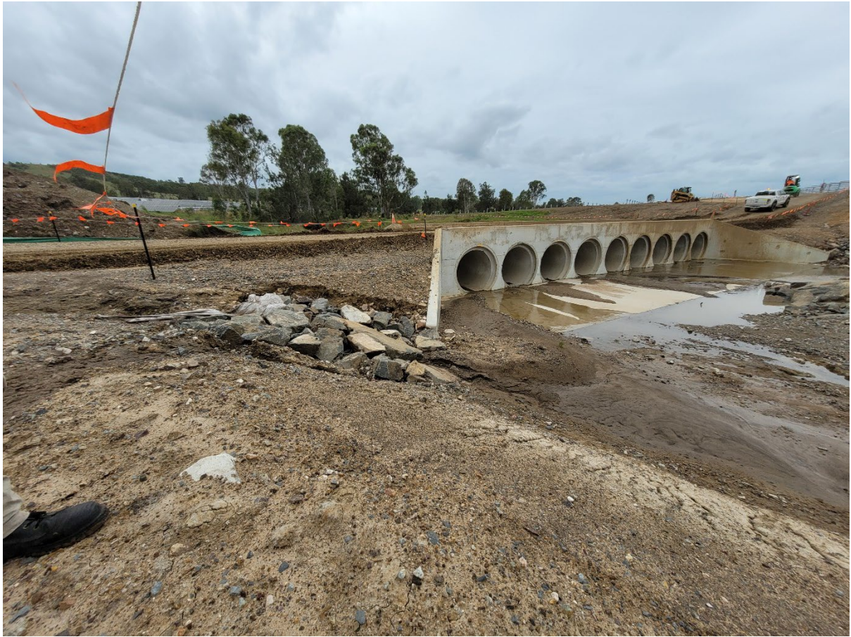
Photo plate 17; an image of washouts filled with rock on the upstream side of culvert 2, taken facing northeast
