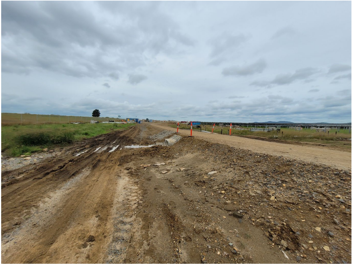
Photo plate 13; an image of culvert 1 taken facing south, showing evidence of vehicle traffic through the waterway, downstream of the culvert
