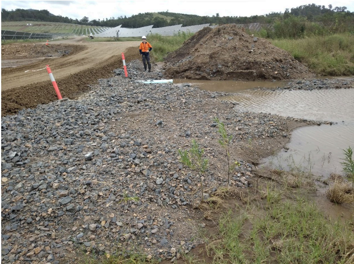
Photo plate 23; an image of the downstream side of culvert 3, showing a pile of fill intersecting the waterway, taken facing north
