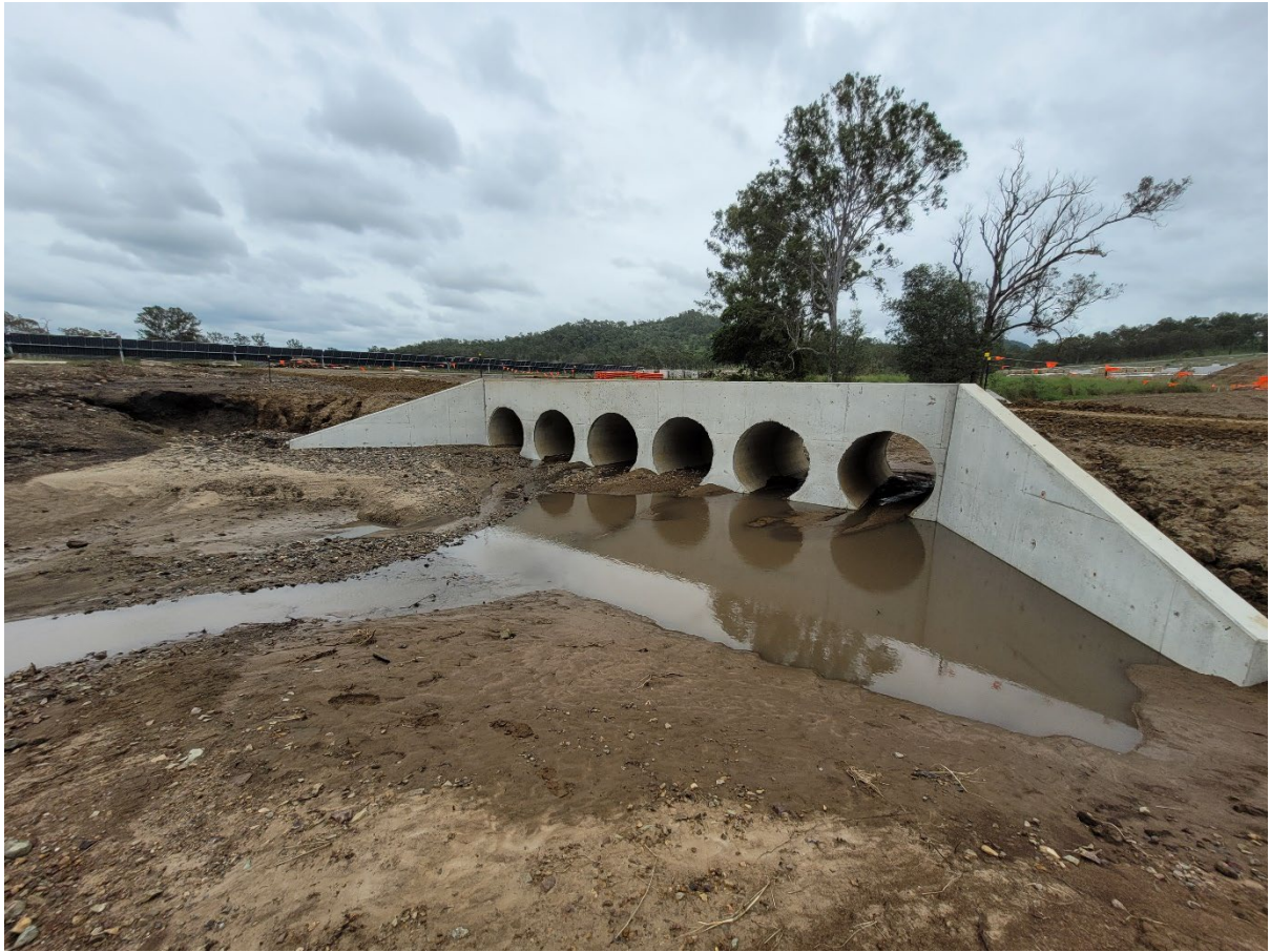
Photo plate 24; An image of the downstream side of culvert 4, showing a washout on the left side of the culvert, taken facing northwest
