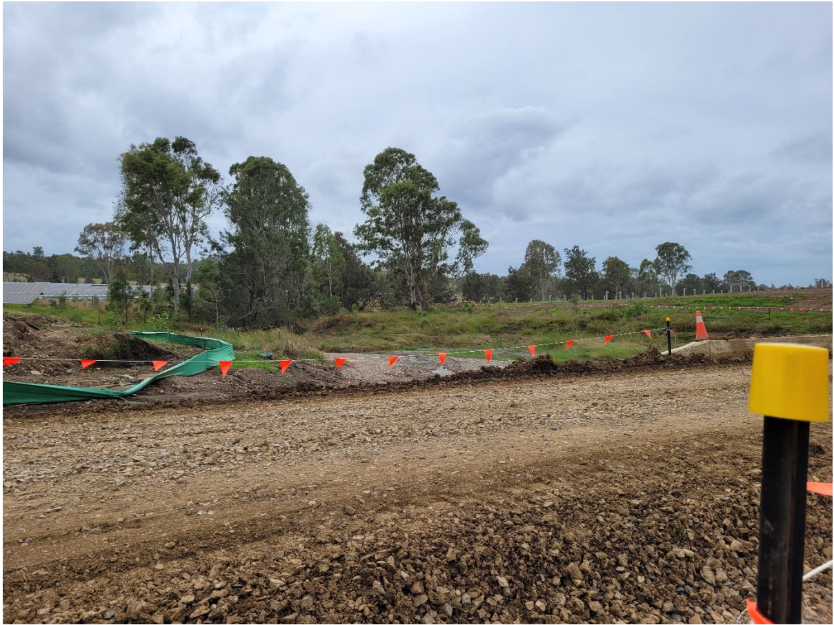
Photo plate 18; shows sediment fencing between a pile of fill and the waterway upstream of culvert 2, taken from the track above culvert 2, facing north
