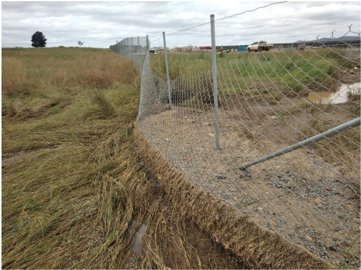
Photo plate 14; an image taken of the eastern boundary downstream of culvert 1, showing sediment build-up against the fence, also a large section of boundary fence without fauna exclusion panelling
