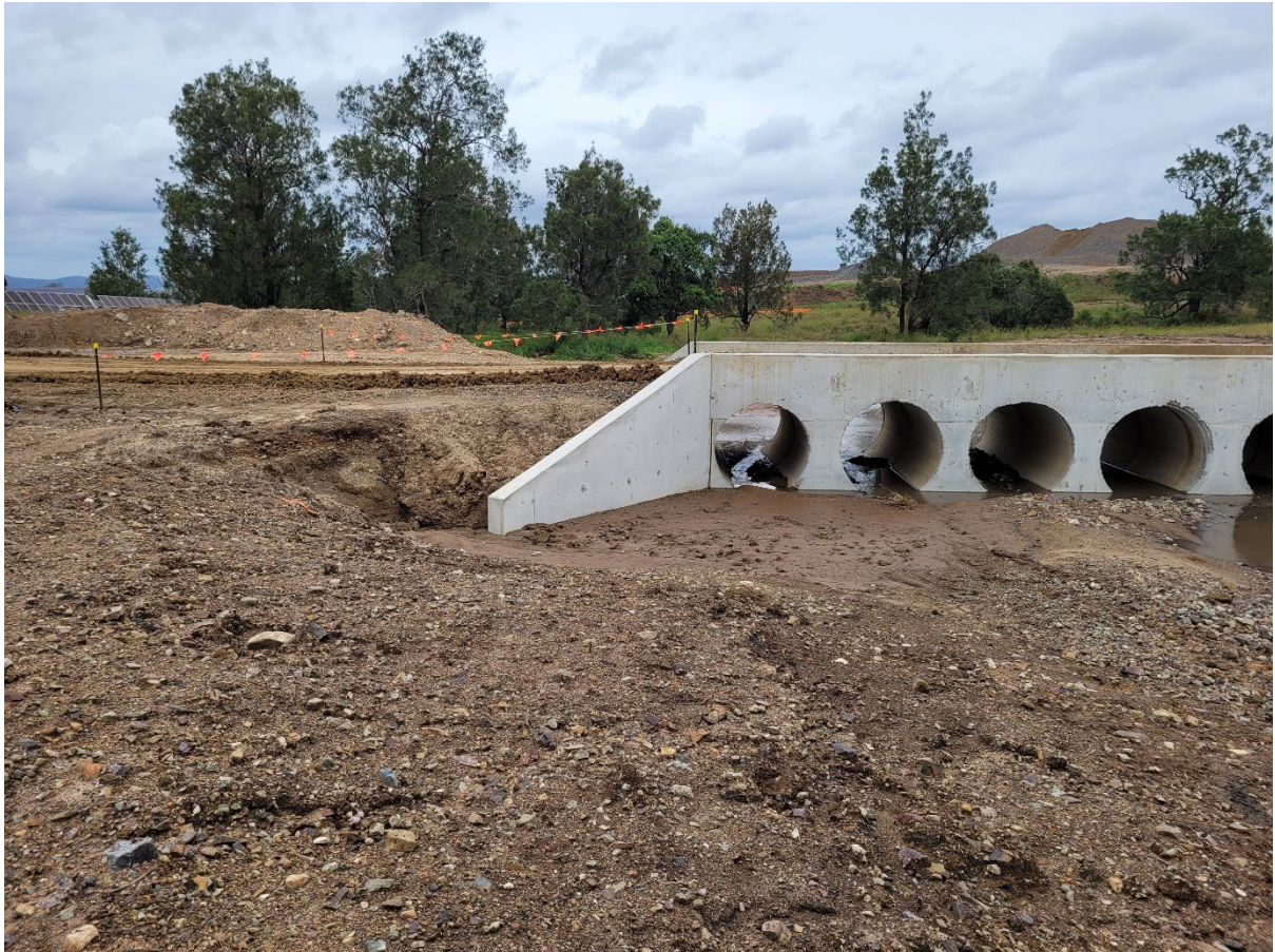
Photo plate 27; an image of the upstream edge of culvert 4, taken facing south, showing a washout on the leftmost side of the culvert
