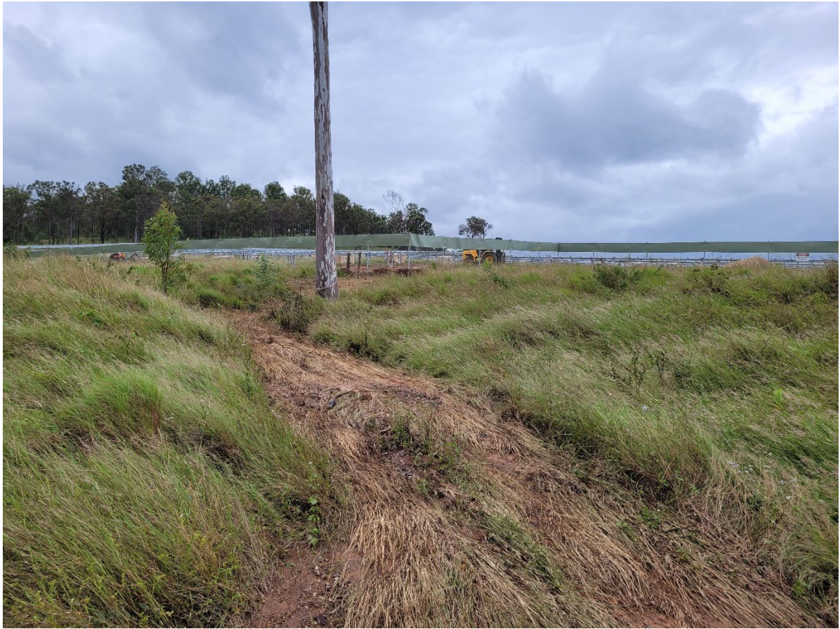
Photo plate 44; a photo showing a channel through which sediment was washed out from the northern boundary through a natural wetland which flowed back into the site, at a GPS location recorded as wash. The photo was taken facing northeast
