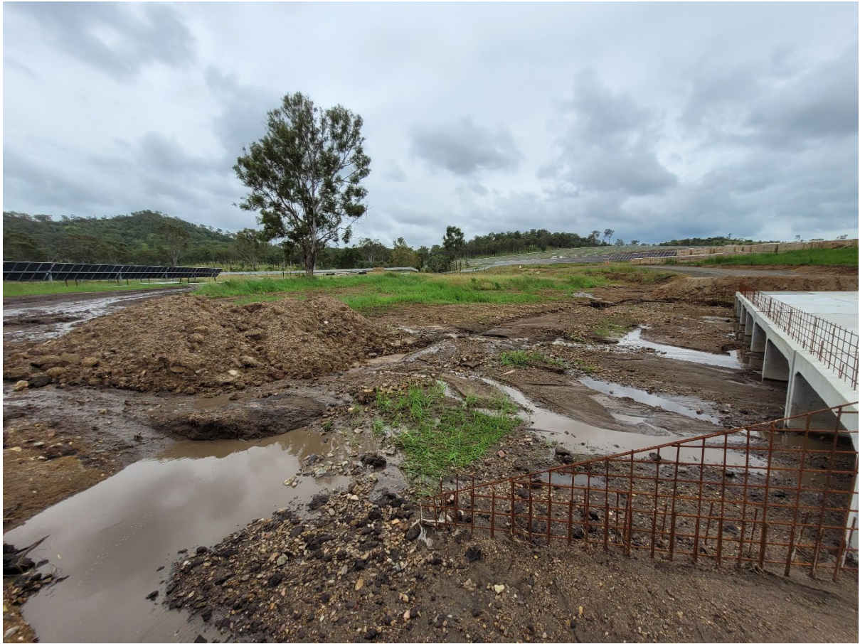
Photo plate 29; a view of the waterway upstream of culvert 5, showing sediment
