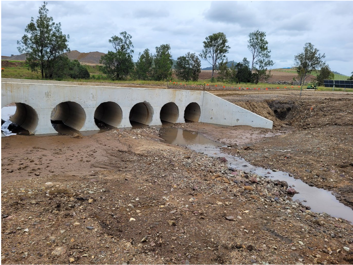
Photo plate 26; an image of the upstream edge of culvert 4, taken facing southwest, showing a washout on the rightmost side of the culvert
